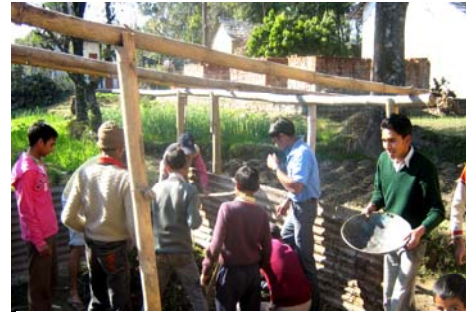
Yuva Mandal Members constructing a toilet
